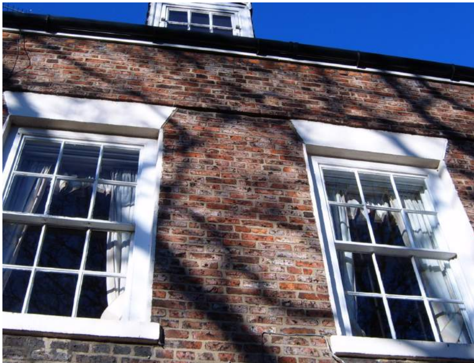
EXAMPLES OF THE EXISTING TIMBER SASH WINDOWS
