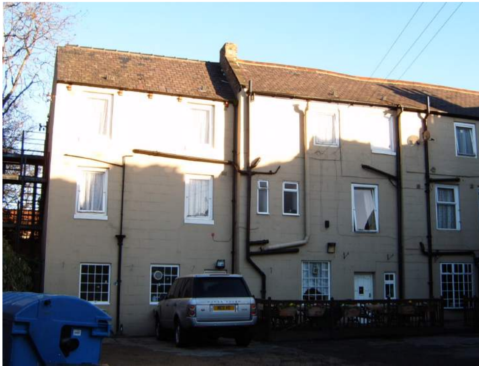
VIEW OF EXISTING WEST ELEVATION FACING INTO THE REAR COURTYARD
